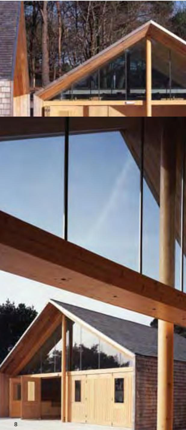
The building envelope was carefully designed with openings placed only within the sheltered gable ends. Sliding folding doors open up fully in summer to provide sheltered spaces with level access from the external decked area, while frameless double glazing above maximizes natural light year round.
