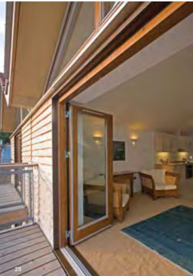
The two wings overlook a new central ecological garden and the river beyond and instead of the small windows used in many green homes, the design incorporates high levels of glazing to maximise daylight and views to the exterior. Externally the terraces are predominantly clad in certified, square edged lapped Western Red Cedar boarding. Cedar was chosen to meet the environmental aspirations of the project and to help the buildings fit within their semi-natural context.
