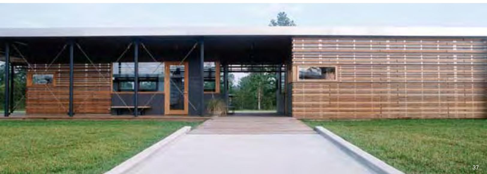
Composed of two volumes connected by a covered breezeway, the southern side of the building is sheltered by a deep overhanging roof, while a translucent polycarbonate northern wall provides ample daylight to interior spaces and allows the building to glow at night. A panelized wood slat screen attached to aluminum straps wraps both the opaque and translucent walls tying together the program elements while adding a degree of warmth and familiarity to the facades.
