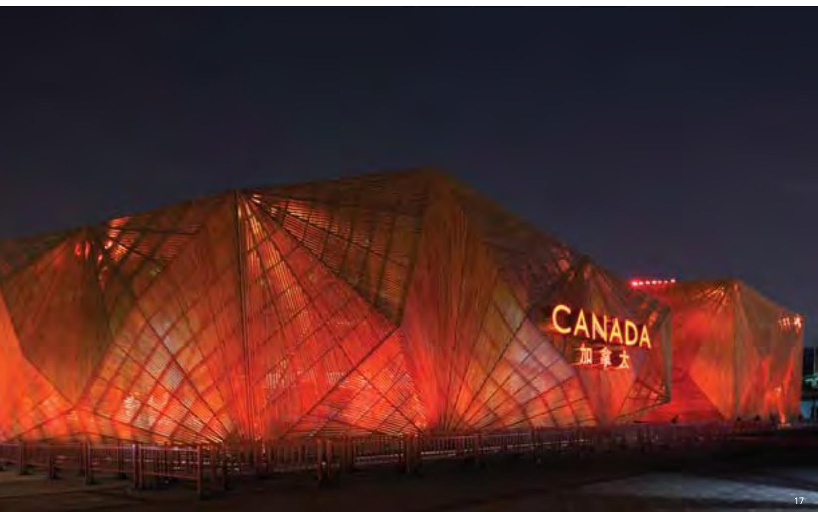
By day the Pavilion is opaque, impressive and imposing, but it undergoes a transformation at night. Lighting mounted on the steel structure behind the cedar skin, glows through the slats giving the pavilion a light, transparent, lantern-like quality.
