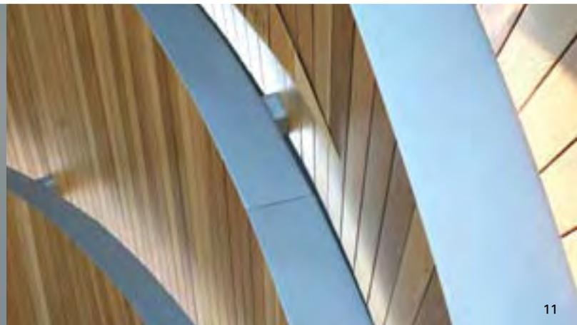
The roof shells were prefabricated off-site, then transported by truck, lifted into place by crane and secured to steel pin connectors cast into the concrete slab. Once installed, the shells were connected with plywood splice plates, and the cedar lining installed.
